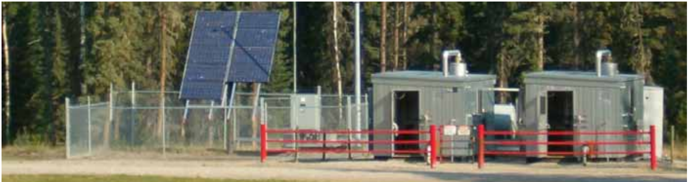
Zero emission wellsite in northeast British Columbia
