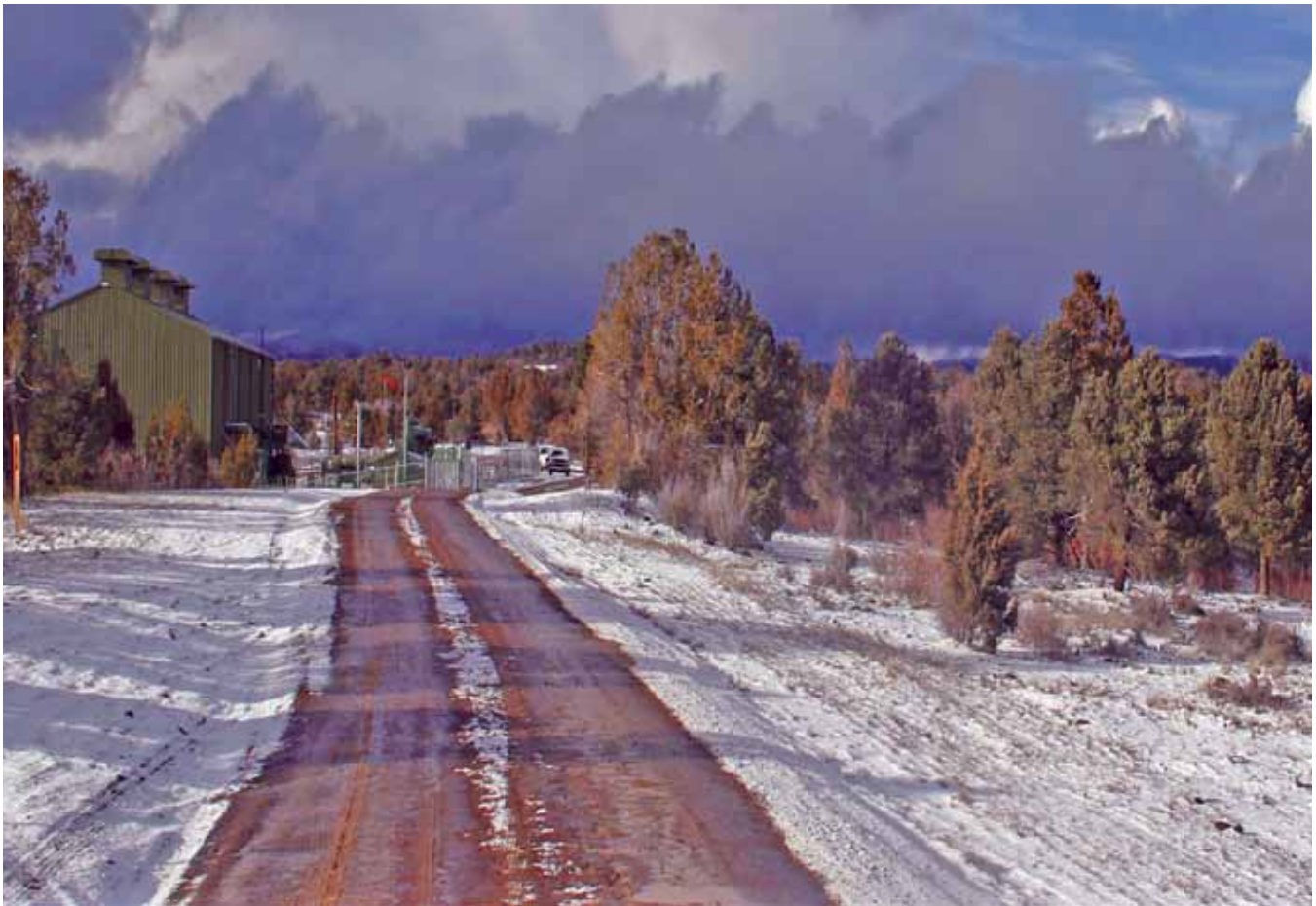
BP San Juan Basin coalbed gas compressor in Colorado
