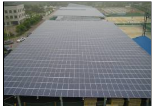
Solar array during construction.
