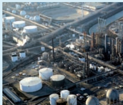
A new 'clean power' plant is proposed adjacent to BP's refinery in Carson, California (left). Petroleum coke – a by-product from refining heavier crude oil – would be processed (as shown above) to produce a synthesis gas stream containing hydrogen and carbon dioxide. The hydrogen would be used to generate electricity, while the carbon dioxide would be captured and sequestered in underground geological formations.
