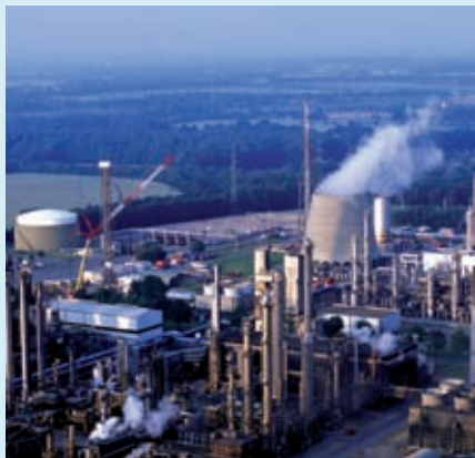
The Veba Combi-Cracking (VCC) process, demonstrated in the 1980s at BP's Gelsenkirchen refinery in Germany (above), could make a comeback for converting heavy hydrocarbons into useful products. The basic VCC process is shown on the right
