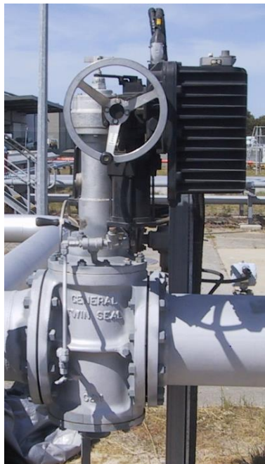
Figure 1: Double block and bleed Valve.
