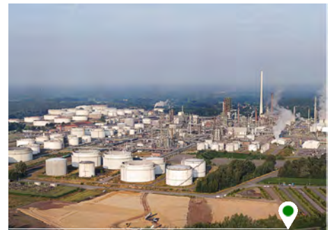
bp's Lingen refinery, Germany
