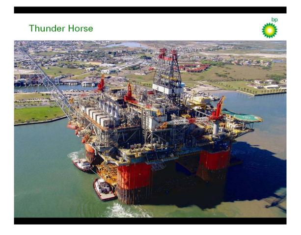
To produce oil from this field BP constructed the largest production semisubmersible ever built. The platform's topside area is the size of three football fields. It contains equipment and systems capable of processing a quarter of a million barrels of oil equivalent per day from over 20 wells. It involved many new technologies and their design, testing and construction required a whole new generation of subsea equipment.
