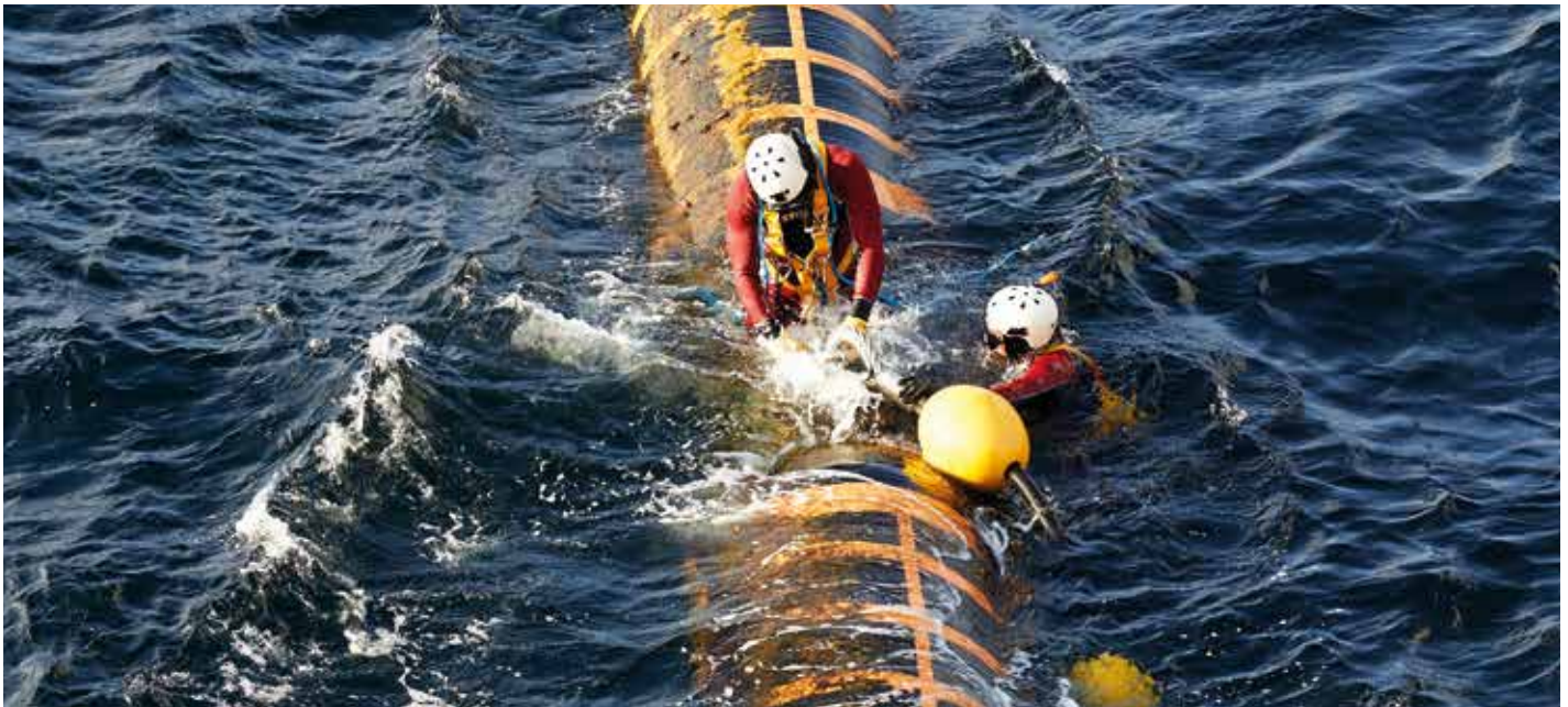
▲ Divers working on the tension hawser cable of the Plutão, Saturno, Vénus and Marte floating production storage offloading vessel (PSVM FPSO).
