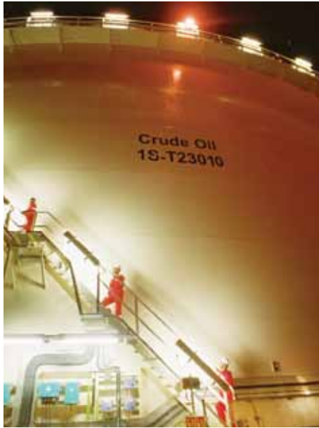
Crude oil tank at Sangachal terminal
