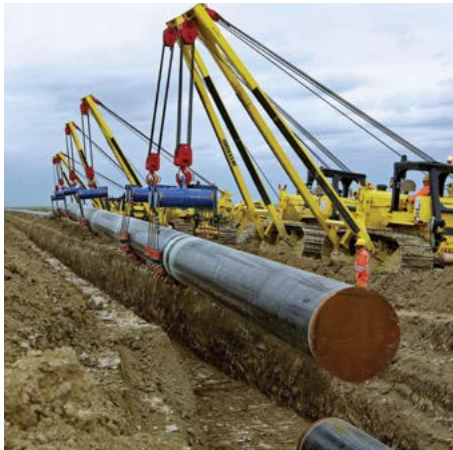
Left: Pipe lowering activity in Hajigabul district as part of the South Caucasus Pipeline expansion project. Right: Construction of Shah Deniz Stage 2 platform topsides is well underway.
