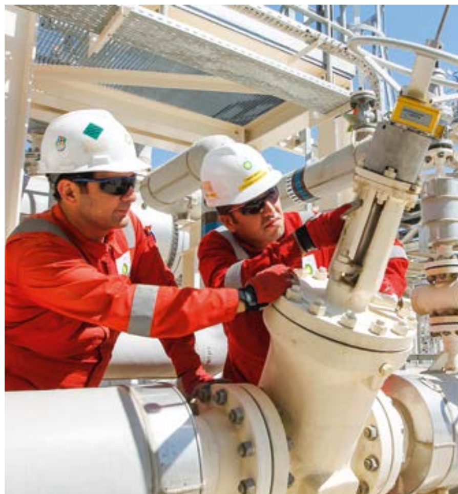
Engineers perform commissioning of an open drains pump as part of the Shah Deniz 2 onshore project activities.
