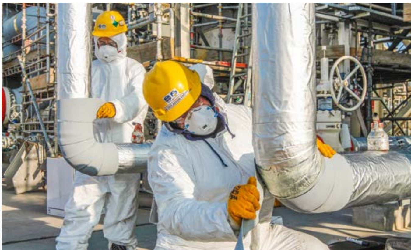
Workers insulate the sections of pipe at the Sangachal terminal.
