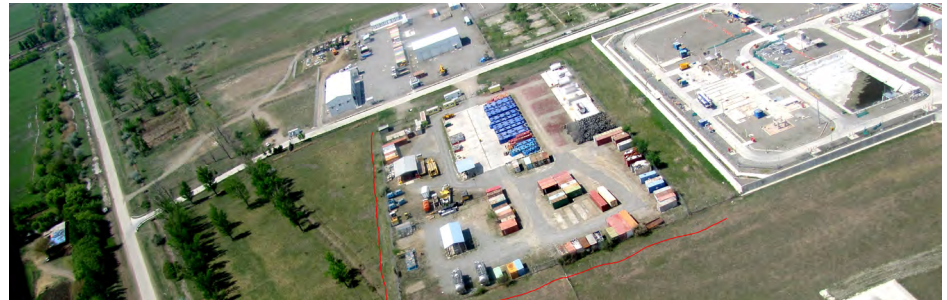
Area for storing waste from BP Georgia sites prior to final disposal.
