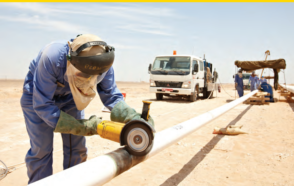
A Dalma welder in protective clothing cuts through piping in Block 61.
