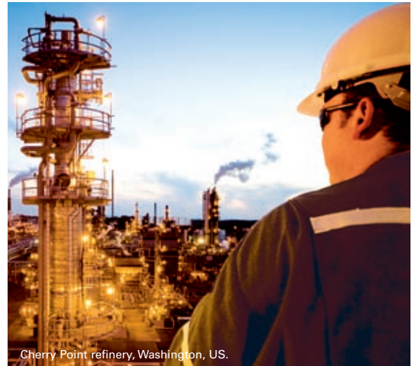
Cherry Point refinery, Washington, US.
