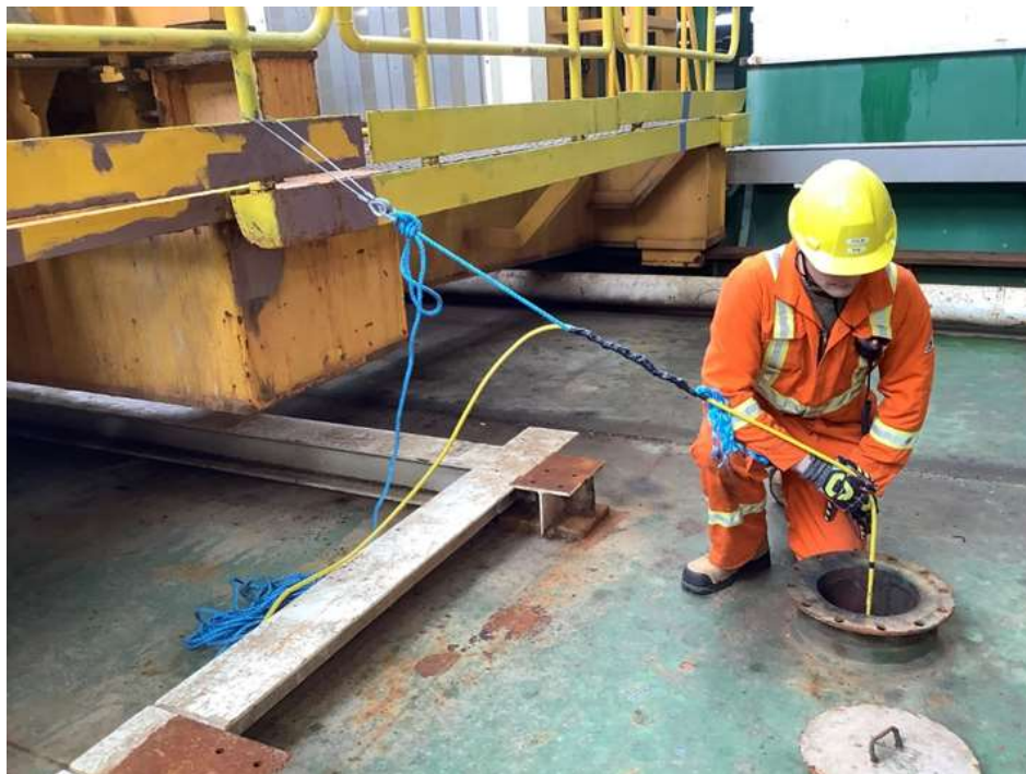
Figure 6-5: Cable Secured to the Rope Using a Chinese Finger Knot (Roman Sandal Tie) to Reduce Cable Tension.
