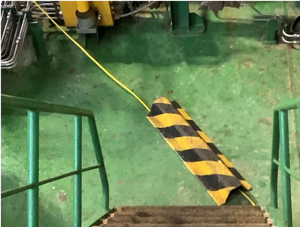
Figure 6-4: Cover to Minimize Cable Damage and Tripping Hazards.
