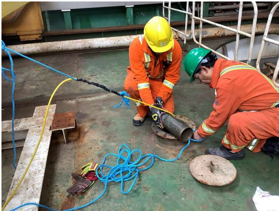
Figure 6-6: Pipe Used to Prevent Cable Abrasion and Keep the Cable Vertical
