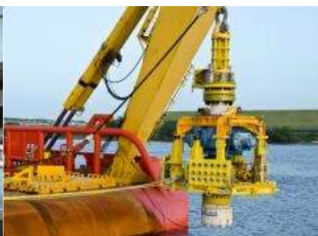
Capping stack installation
