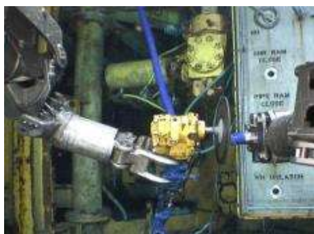
Direct intervention on BOP
