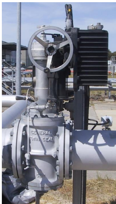
Figure 1: Double block and bleed Valve.
