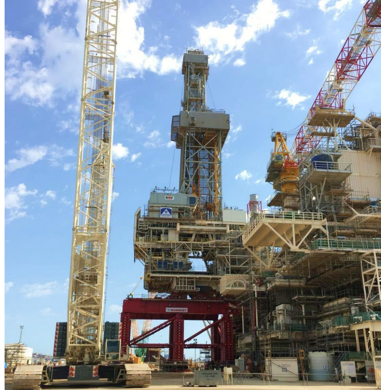
Drilling facilities 'Jack and Skid' operation at Bibi-Heybat yard
