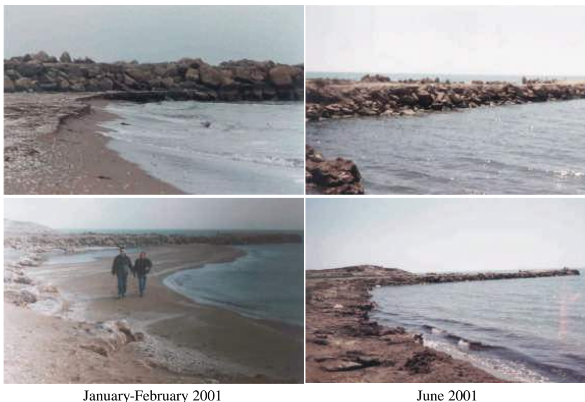
Figure 6.26 Erosion at base of jetty – western side
