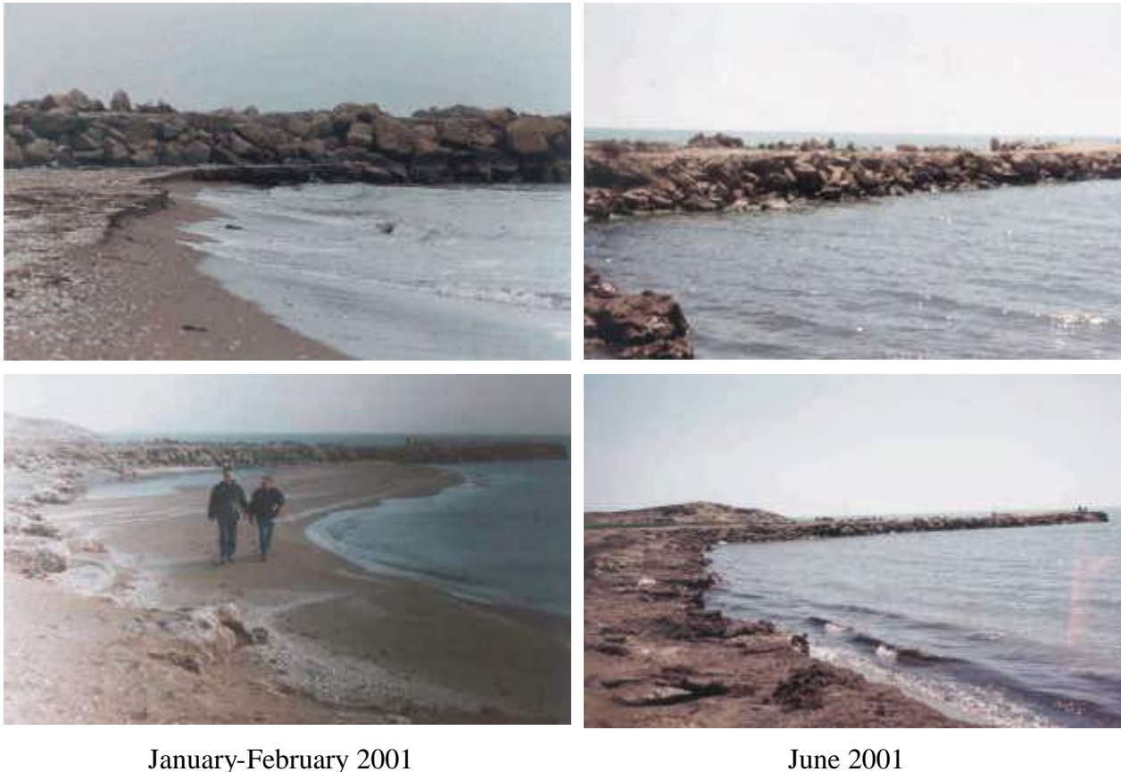
Figure 12 Erosion at base of jetty – western side
