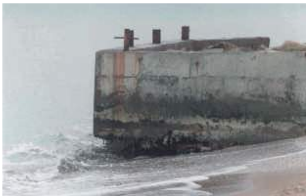
Figure 11 Erosion at base of jetty – eastern side
