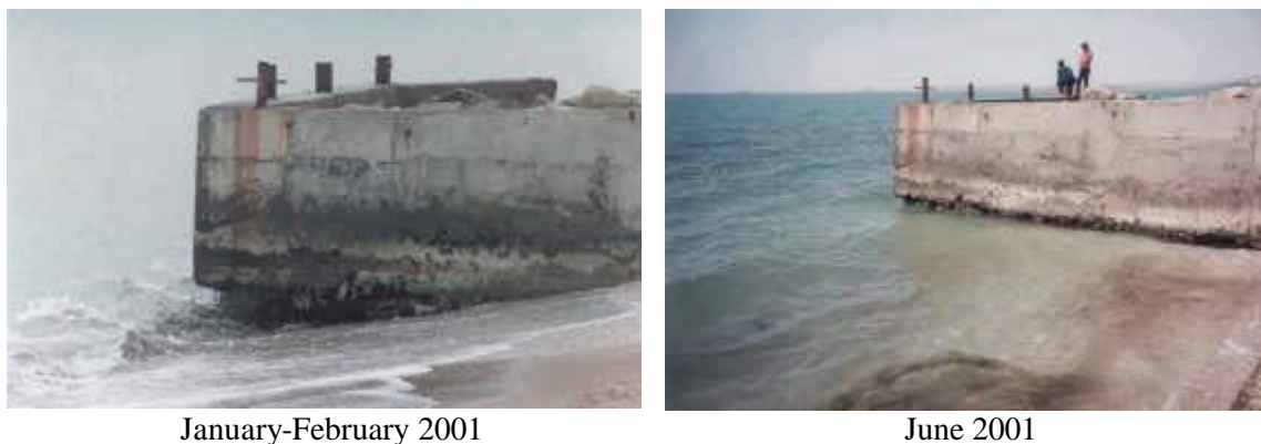
Figure 6.25 Erosion at base of jetty – eastern side
