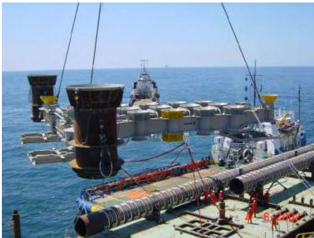
Figure 0.7: Installation of the Phase 1 Drilling Template
