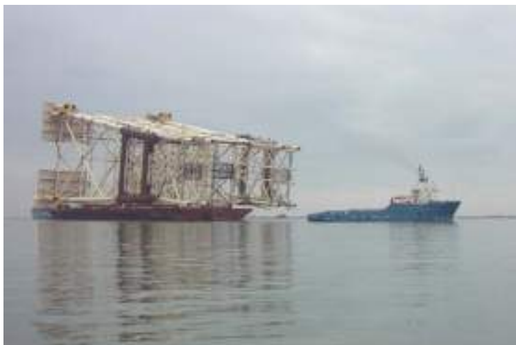
Figure 5.14 Jacket Tow Out
