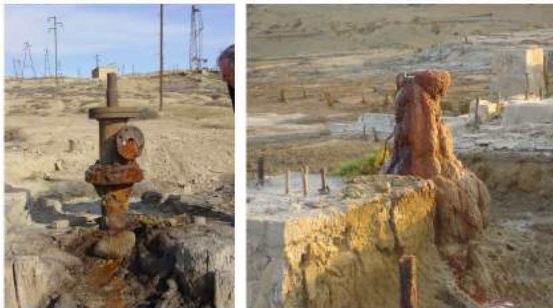
Figure 4.5 Photograph of leaking wellheads at Lokbatan
