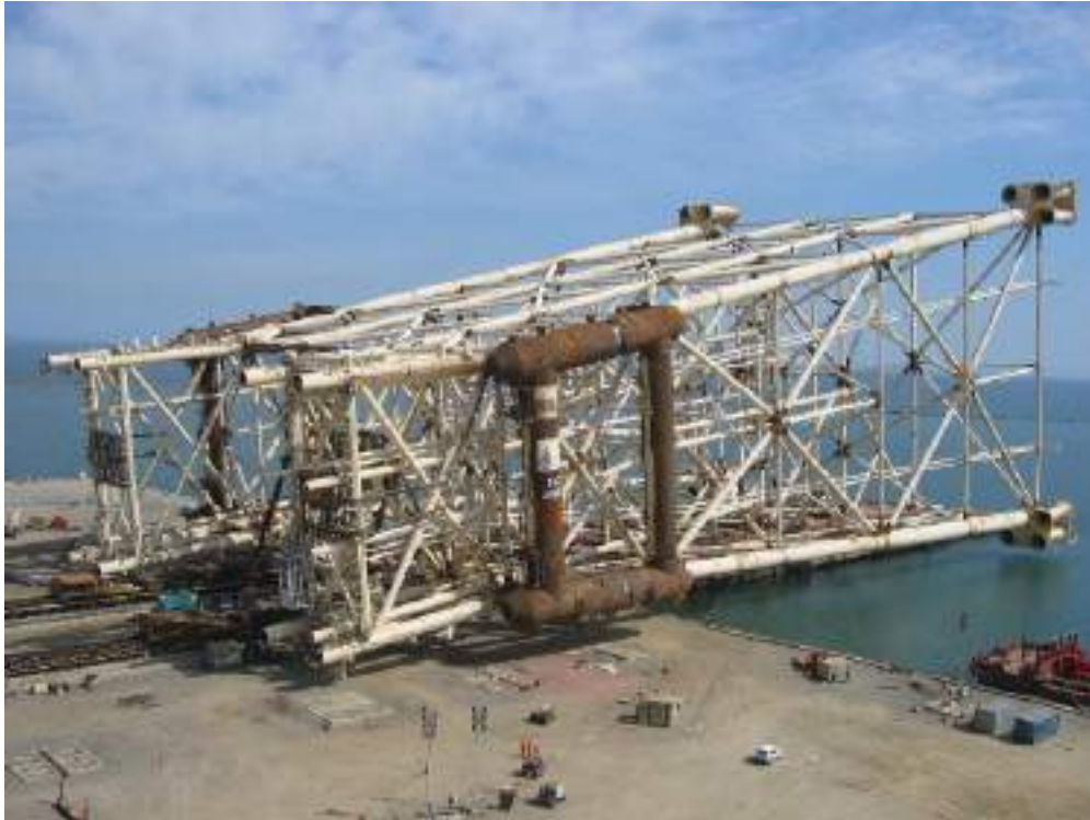
Figure 5.10 DWG-DUQ Jacket During Loadout
