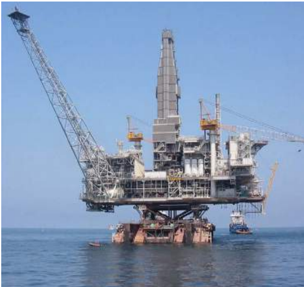
Figure 5.11 EA Platform Topside Onboard STB-1 Barge
