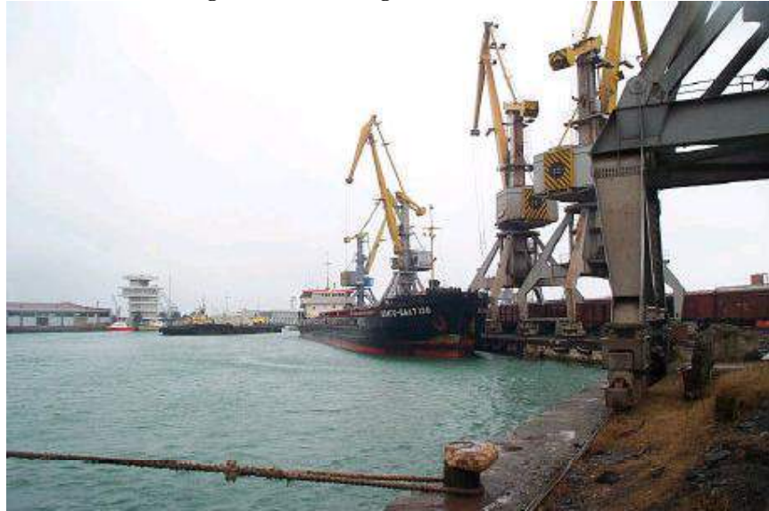
Figure 5-8 Unloading facilities at Poti Port
