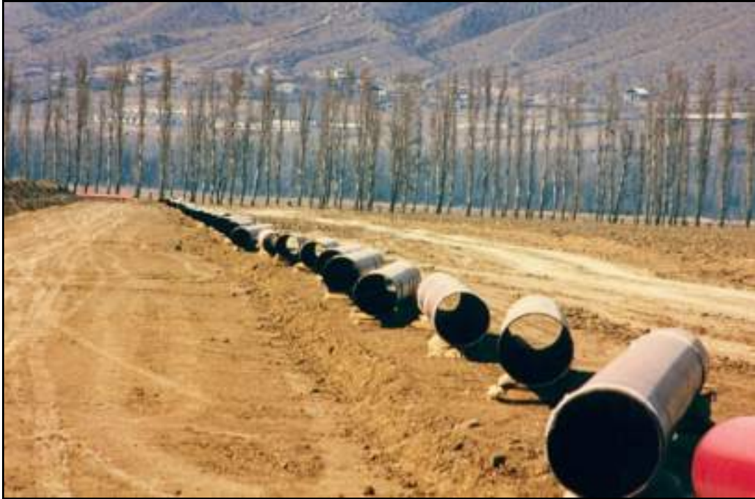
Plate 4.1 Photograph of a Pipe Stringing along the RoW
