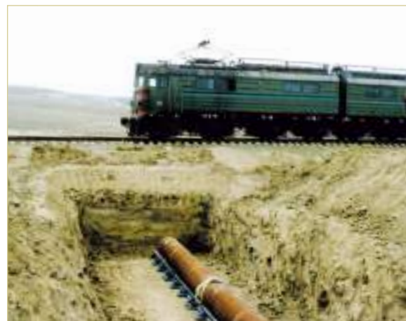
Pipeline passing beneath railway line
