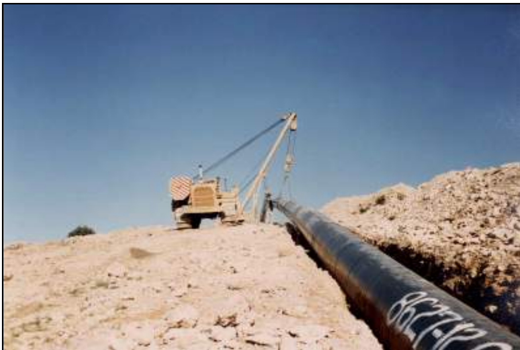
Plate 4.3 Photograph of Laying a Pipe into a Trench [Source: ILF]
