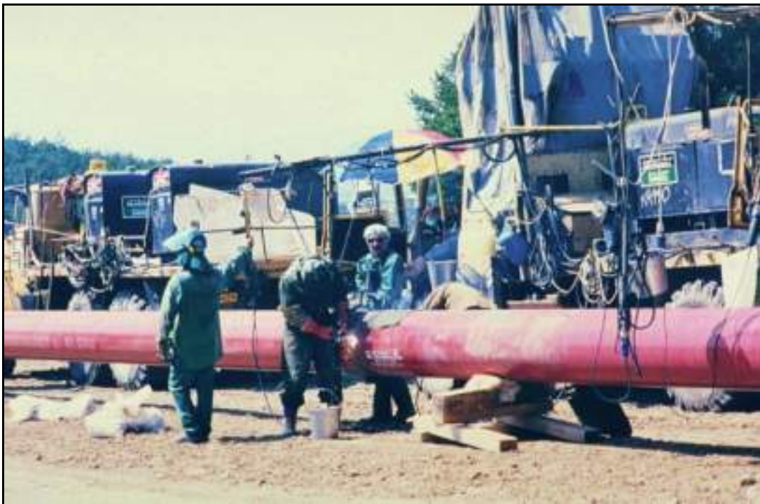
Plate 4.2 Photograph of Pipe Welding Operations
