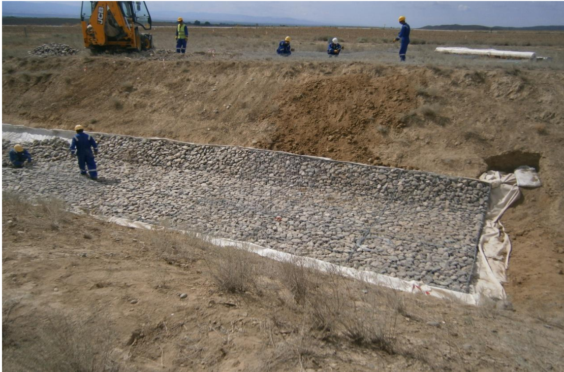
Figure 2.5: Gabions on River Crossing at KP 419.2
