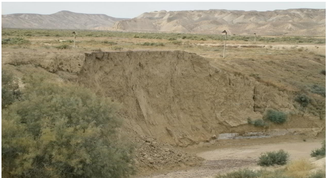
Figure 2.2: Erosion at Djeyrankechmez River crossing
