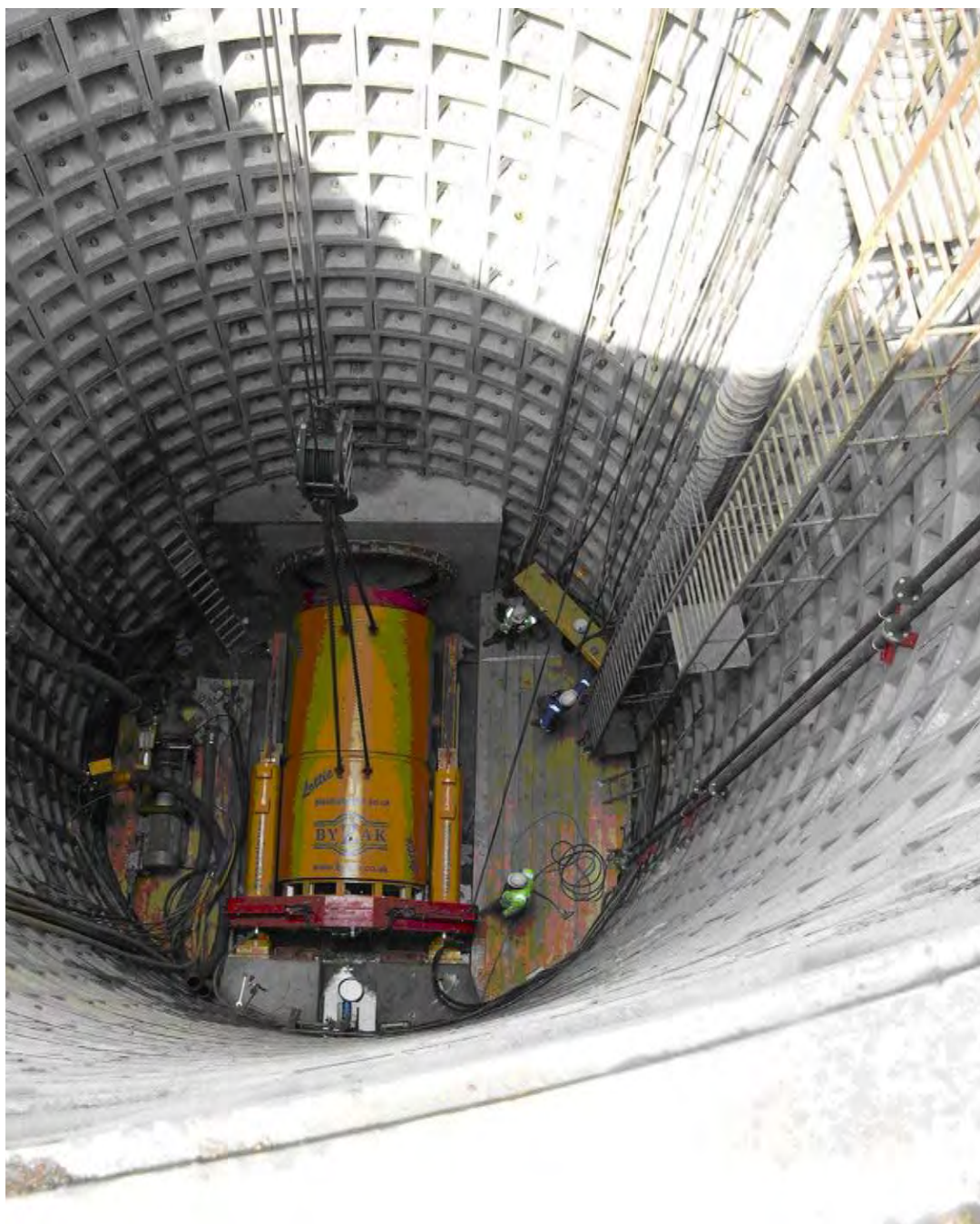
Figure 5-20: Jacking Frame in a Launch Pit
