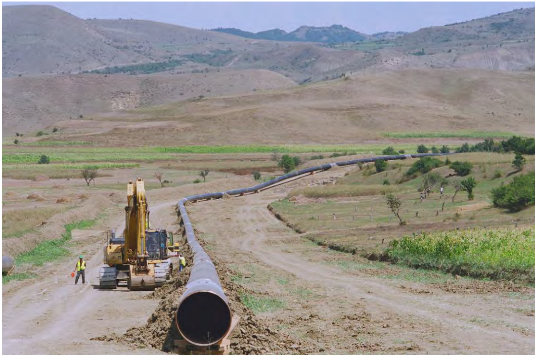
Figure 5-16: Pipeline Welded Together
