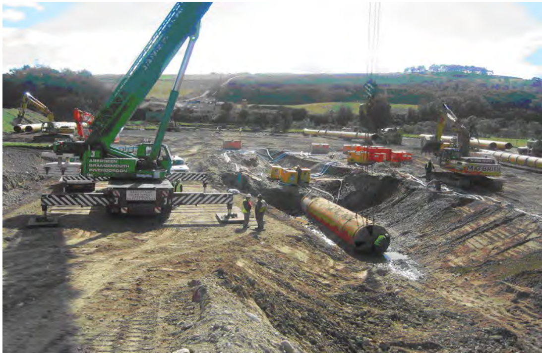
Figure 5-21: TBM at a Reception Pit
