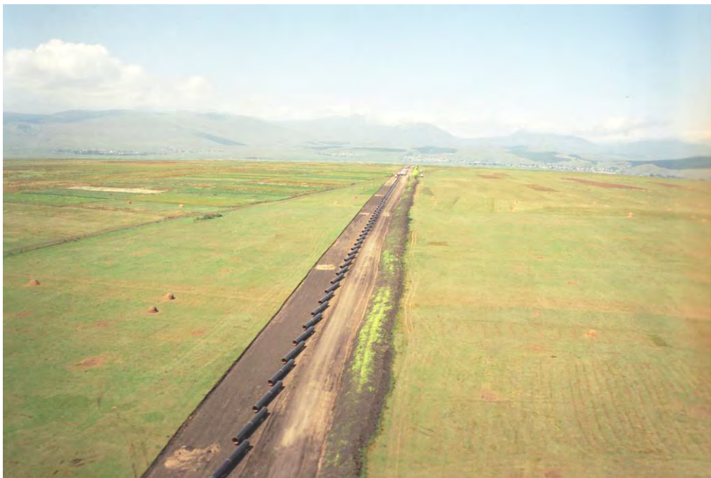
Figure 5-15: Topsoil-Stripped ROW and Pipeline String Ready for Welding
