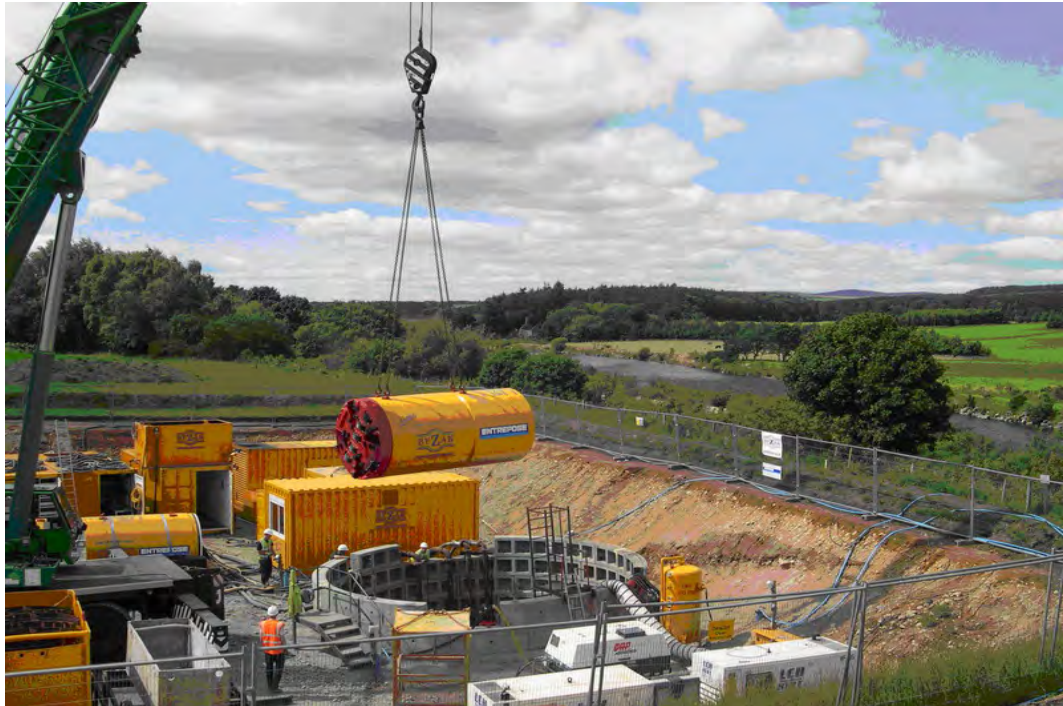
Figure 5-19: TBM Being Lowered into a Launch Pit
