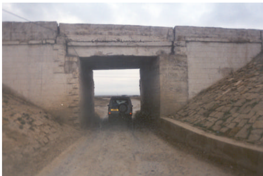
Figure 8-25 Typical railway underpass
