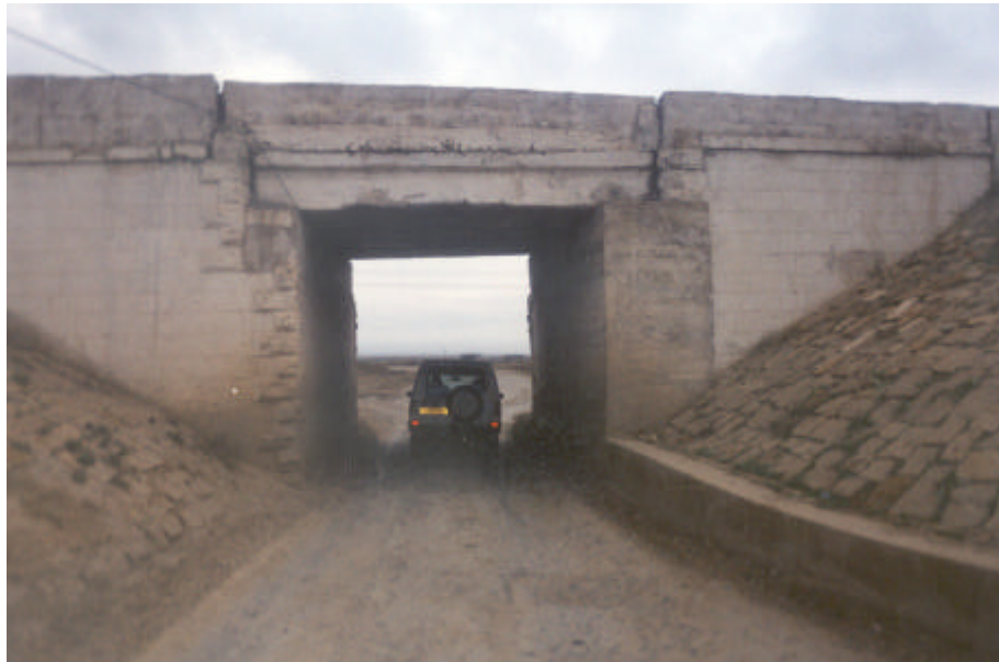
Figure 1 Typical railway underpass
