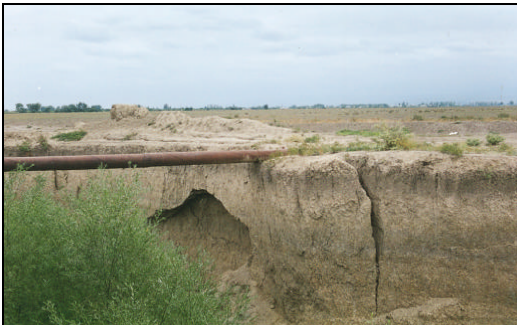
Figure 7 Extensive bank erosion at a branch of the Ganjachay River (KP 295)
