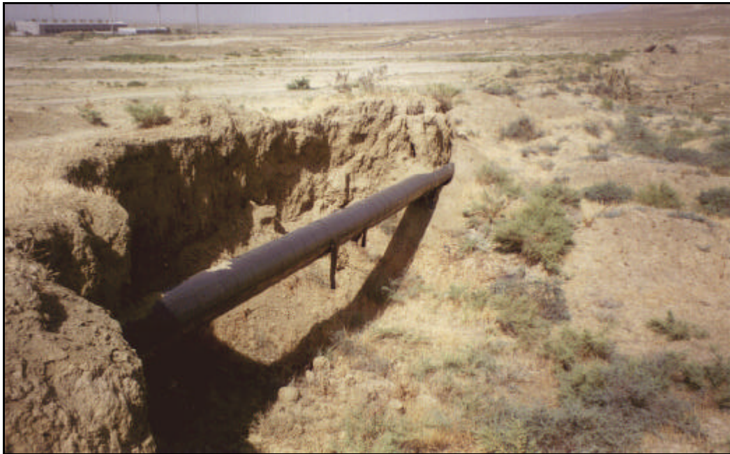
Figure 9 Pipe exposed by erosion in wadi
