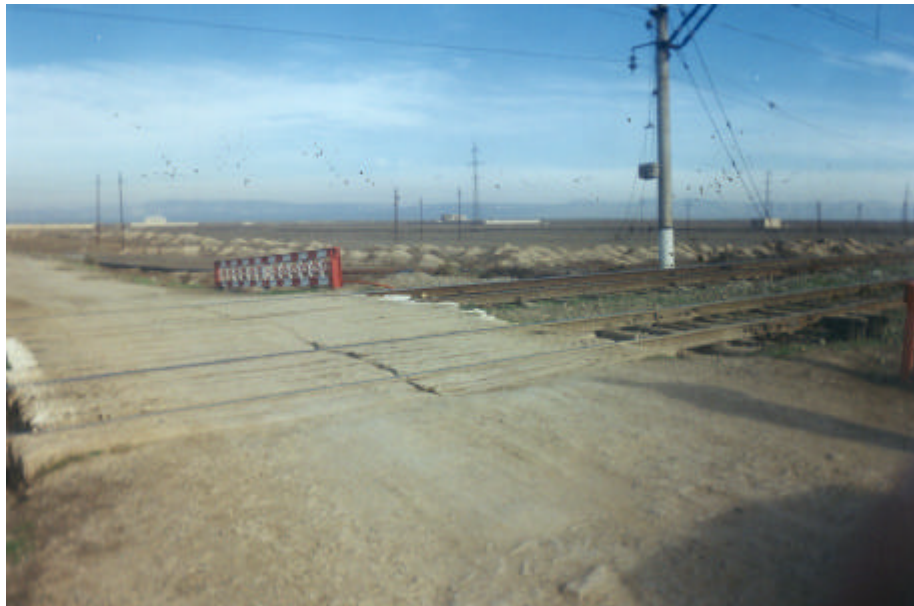
Figure 2 Typical railway crossing without bridge
