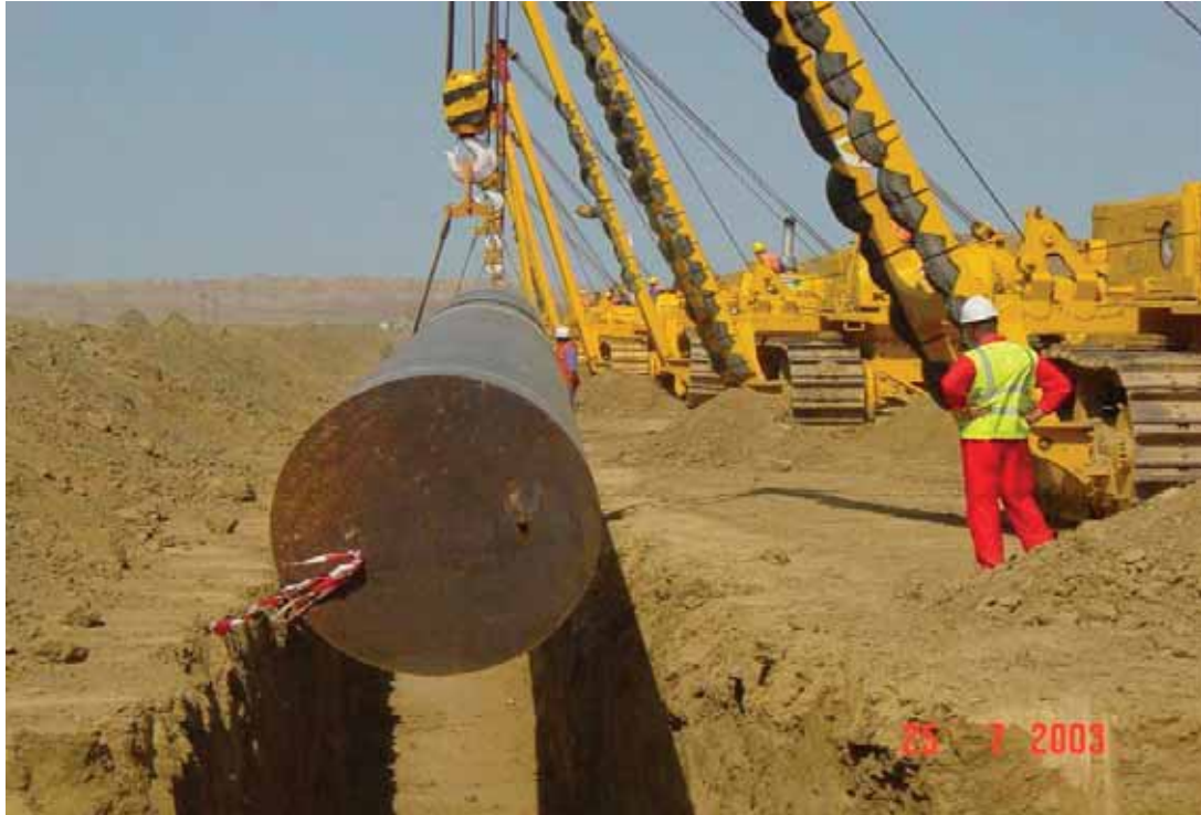
Photograph 5-4: Lowering-in of the Pipeline
