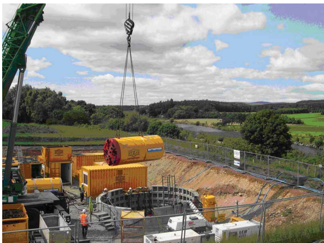
Photograph 5-5: Micro-tunnelling Beneath a River
