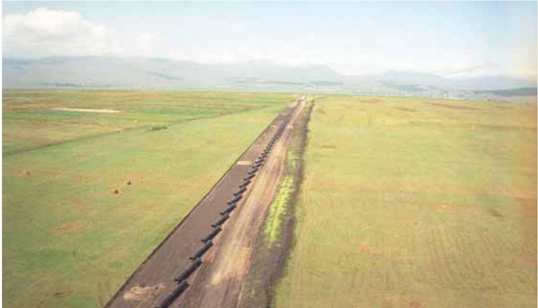
Photograph 5-2: Topsoil-Stripped ROW and Pipeline String Ready for Welding
