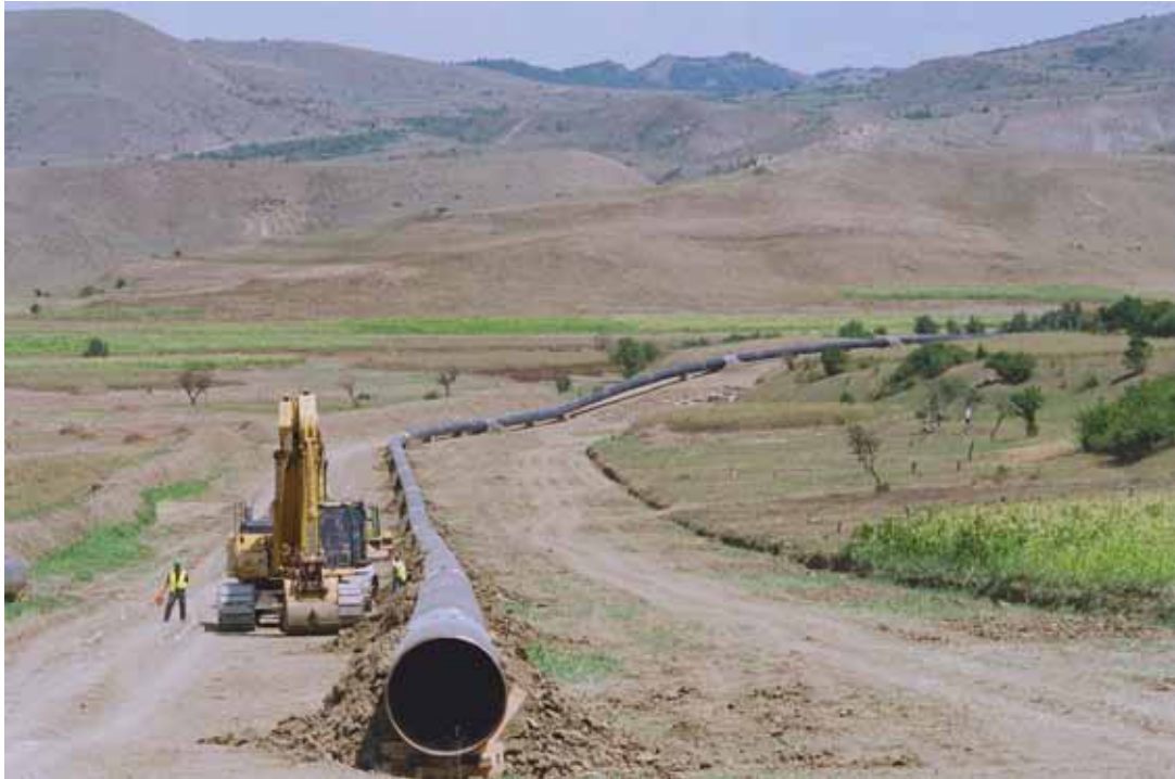
Photograph 5-3: Welded Pipeline
