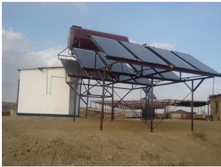
Solar batteries for the water heater in Eyvazlar farm
