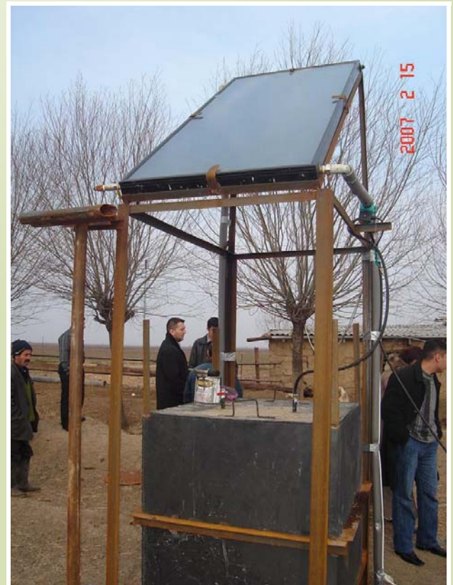
Biogaz unit with solar panel
