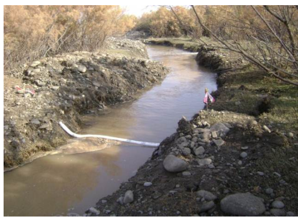
Before: Turbid water entering the main watercourse
