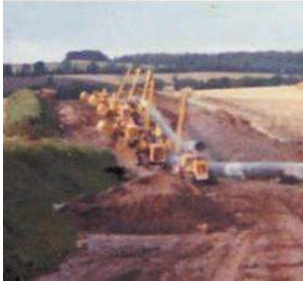
Figure 5.33 Typical spread and side -boom
