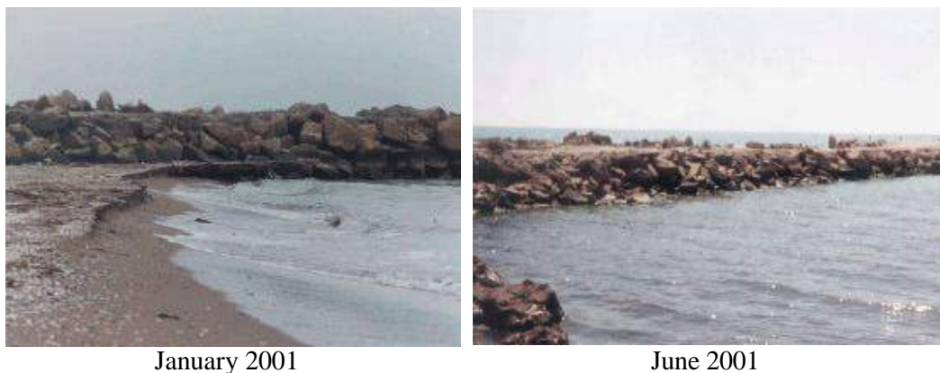
Figure 6.28b Erosion at base of jetty - western side
