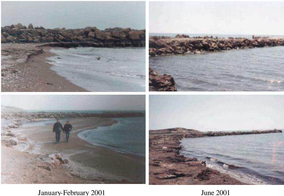
Figure 12 Erosion at base of jetty – western side
