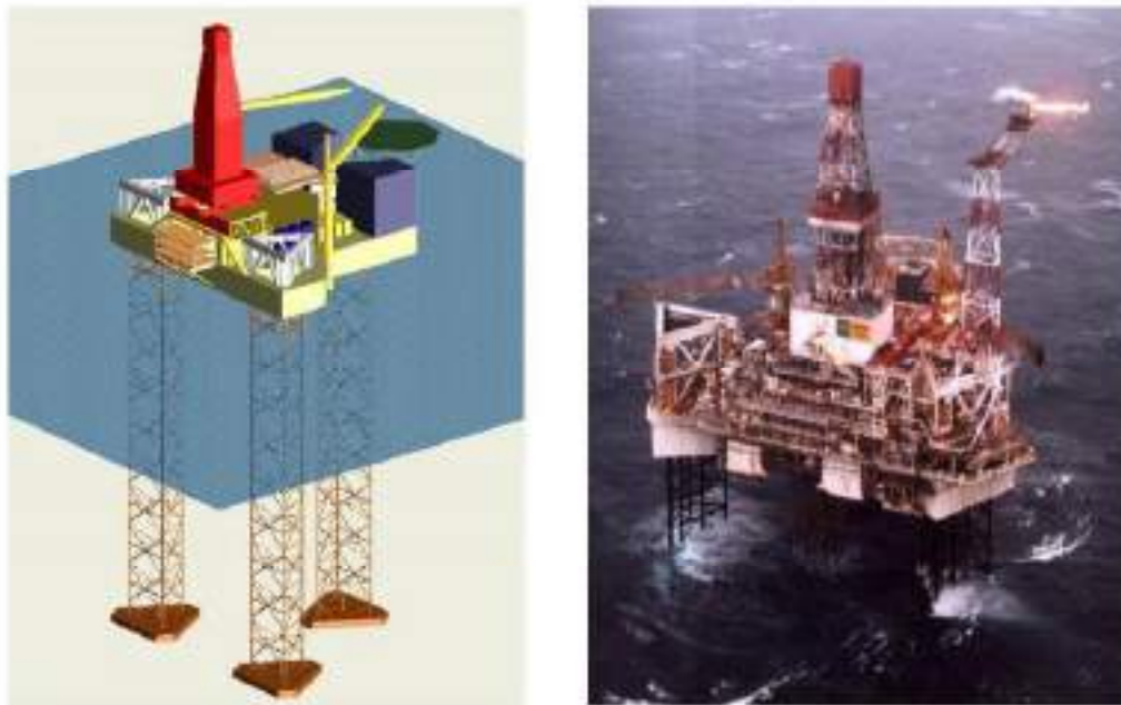
Figure 5.12 The self-installing TPG500 (proprietary) drilling rig
