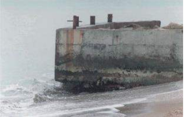
Figure 11 Erosion at base of jetty – eastern side
