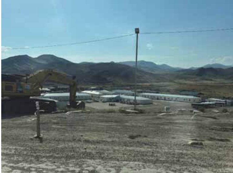
Figure 5.29: Temporary accommodation for motorway construction workforce
