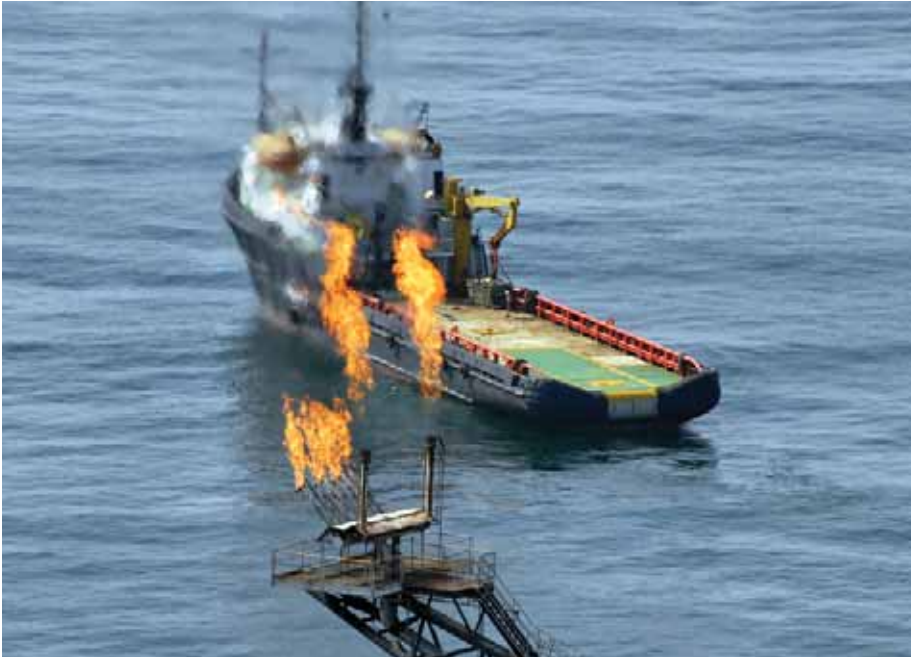
Flaring at Chirag platform
