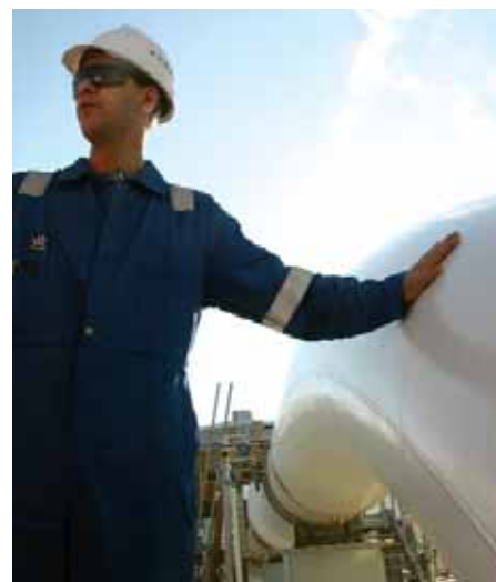
BTC pipeline starts here - at Sangachal terminal.
