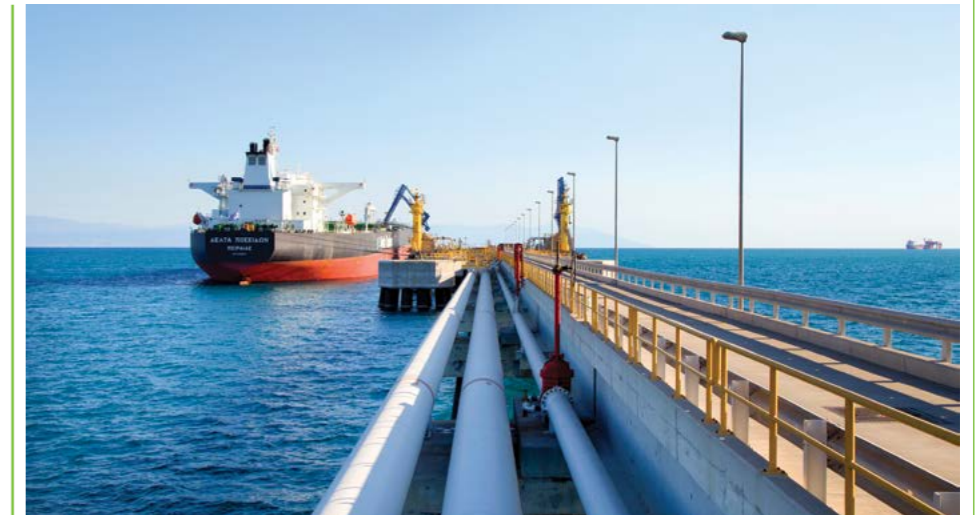
Tanker loading process at Ceyhan Marine terminal jetty.
