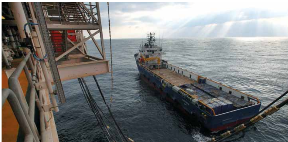
Supply vessel at East Azeri platform.
