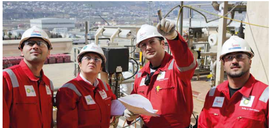
Our employees at the West Chirag topside construction site.
