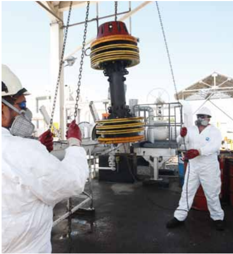
Technicians conducting routine pig launch operation at a pump station.
