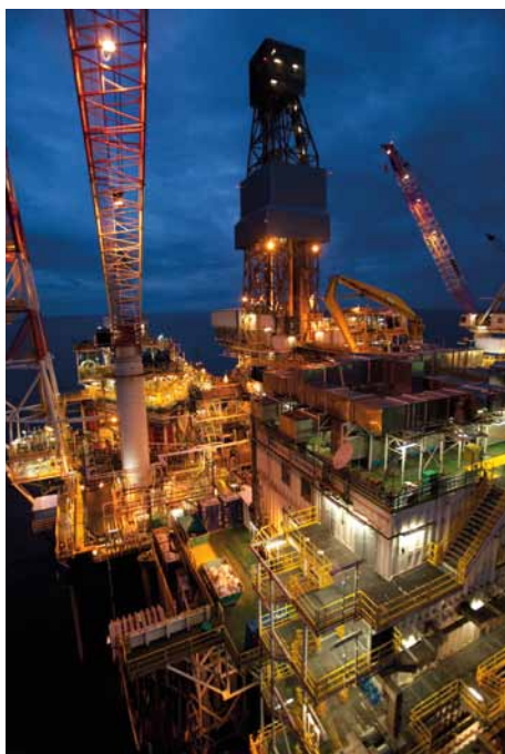
Night view at Shah Deniz platform.
