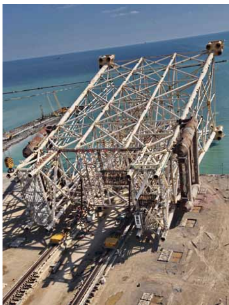
West Chirag platform jacket being loaded onto the transportation barge.
