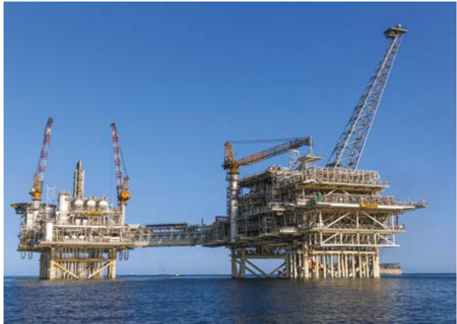
Shah Deniz Bravo platform successfully installed offshore.
