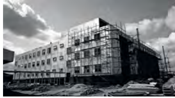
Construction of new Aberdeen headquarters in 1973.
