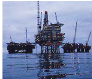
Miller platform with flotels Safe Britannia and Safe Holmia.
