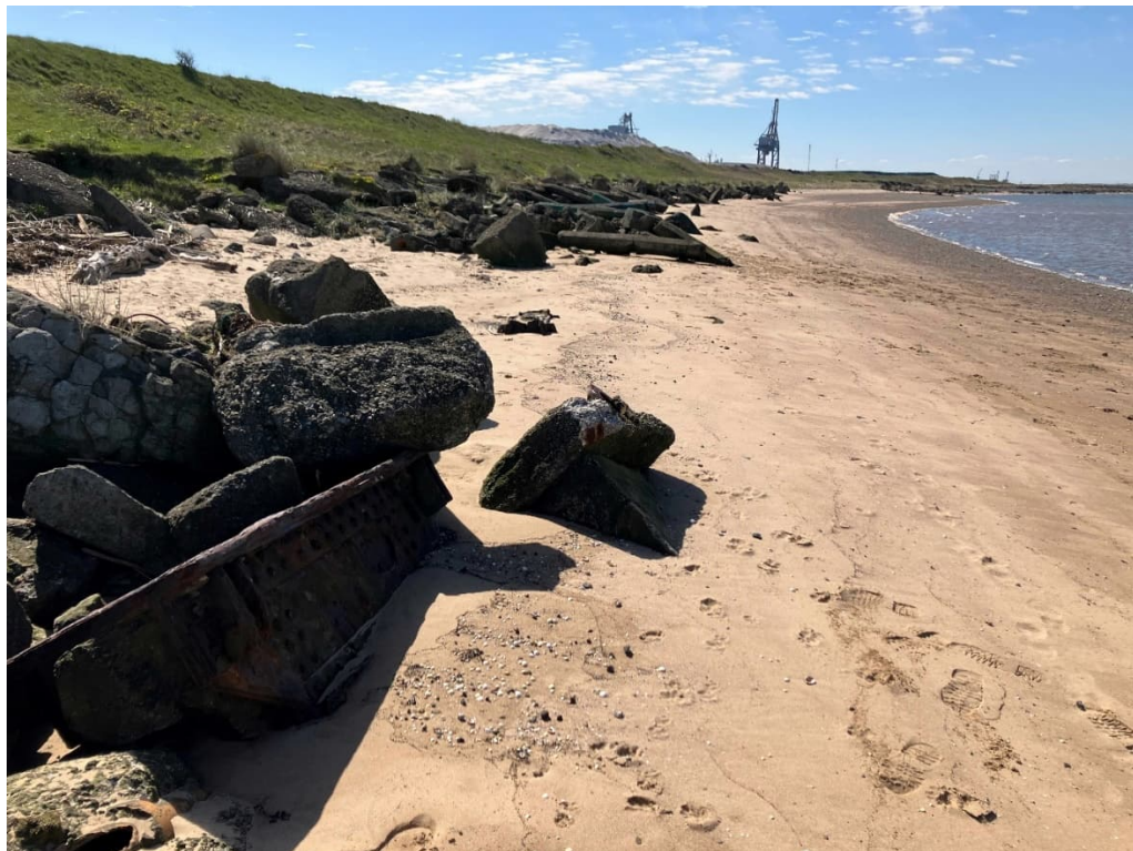
Plate 17A-12: View south-west along the edge of Bran Sands, showing battered edge of made ground underlying Redcar Bulk Terminal
