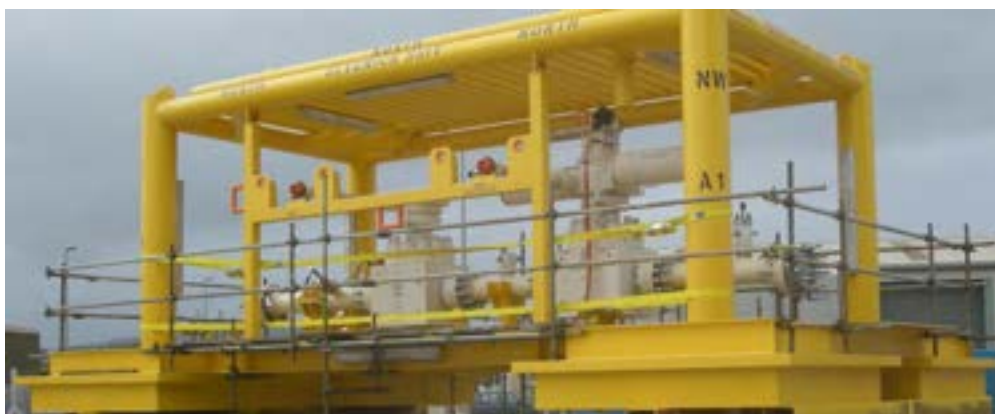
Figure 3-9 - Typical SSIV structure, analogous to that to be installed on the Teesside Pipeline
