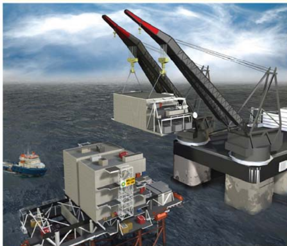
Power generation module being lifted by heavy lift vessel.
