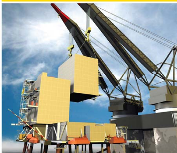
Gas process module being lifted by heavy lift vessel.
