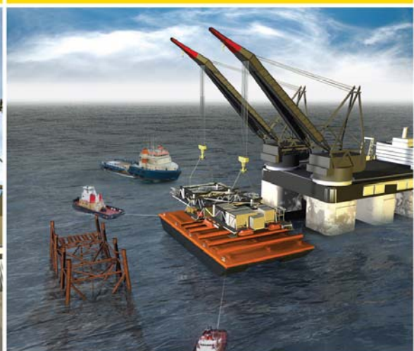
Module support frame being placed on a transportation barge.
