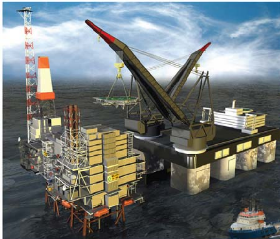
Heavy lift vessel lifting the helideck.
