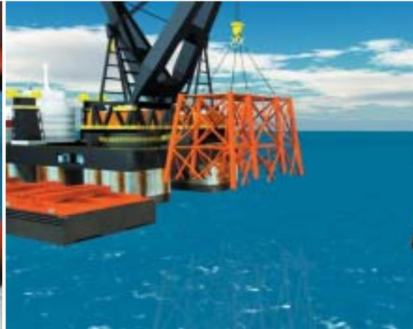
**2** Top section of the jacket being lifted by a heavy lift vessel to be placed onto a transportation barge
