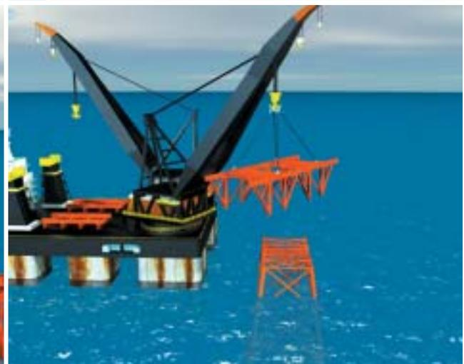
6 Module support frame being lifted by heavy lift vessel
