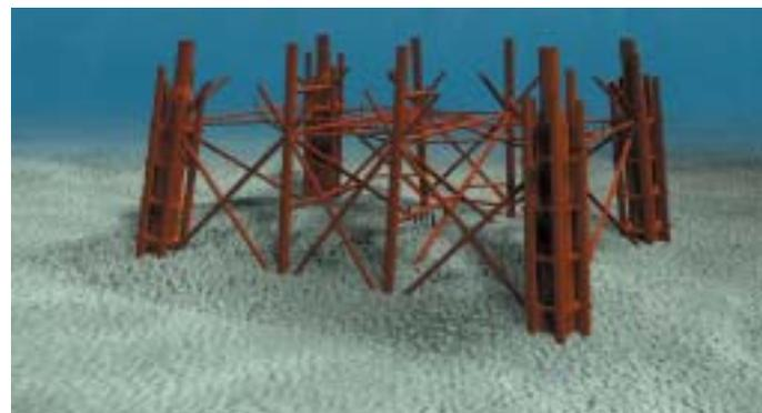
**Figure 8.3c:** Computer graphic of the North West Hutton support structure after removal of the upper jacket to the top of the footings.
