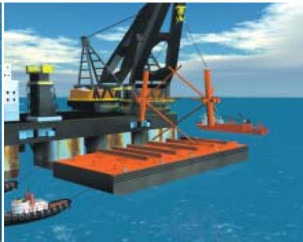
**4** Jacket section being lowered onto a barge for transportation to the shore for disposal
