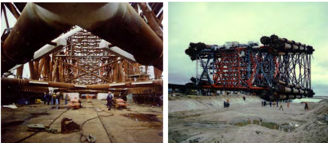
Photographs courtesy of Charles Hodge, Lowestoft, Norfolk Figure 2.7: Photographs of the North West Hutton Jacket
