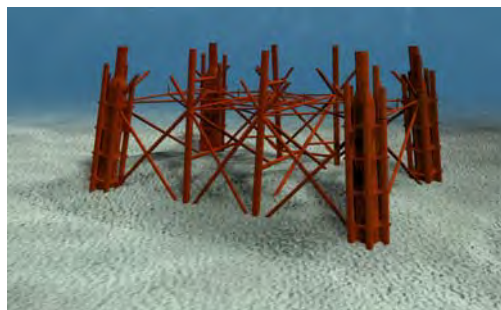
Figure 8.3c: Computer graphic of the North West Hutton support structure after removal of the upper jacket to the top of the footings.
