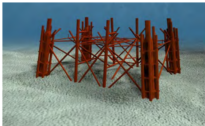
Figure 2.8: Computer graphic of the North West Hutton support structure after removal to the top of the footings
