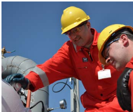
Equipment maintenance Baku-Tbilisi-Ceyhan Pump Station 1
