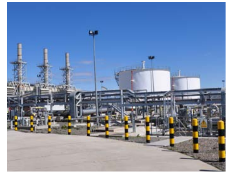
Operating facility Baku-Tbilisi-Ceyhan Pump Station 1
