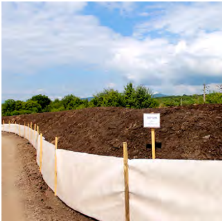
Temporary storage of topsoil at a construction site.
