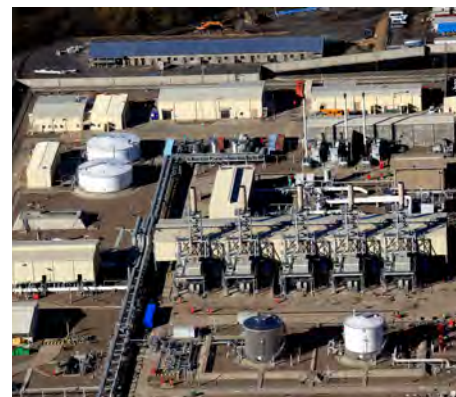
Aerial view of BTC pump station 2.
