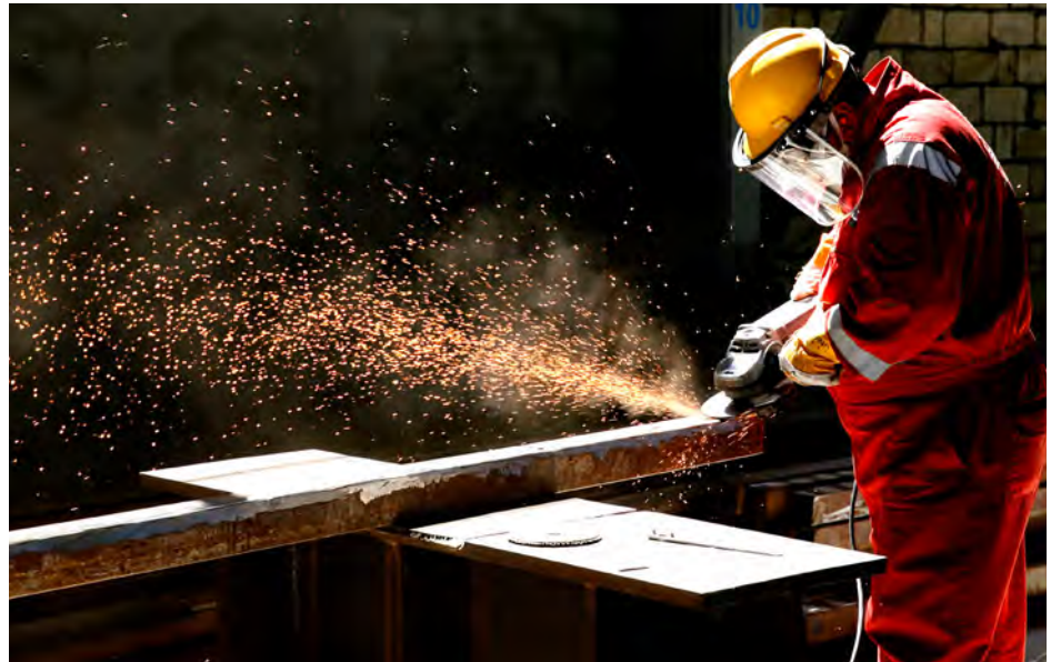
▲ An employee performing maintenance work at site.
