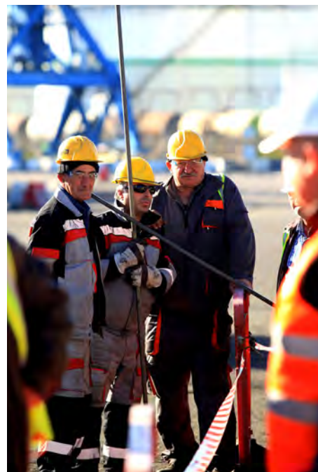
People at work at pipes receiving location.
