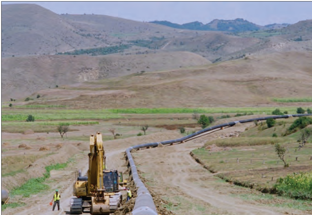
Figure 5-4: Welded Pipe Section
