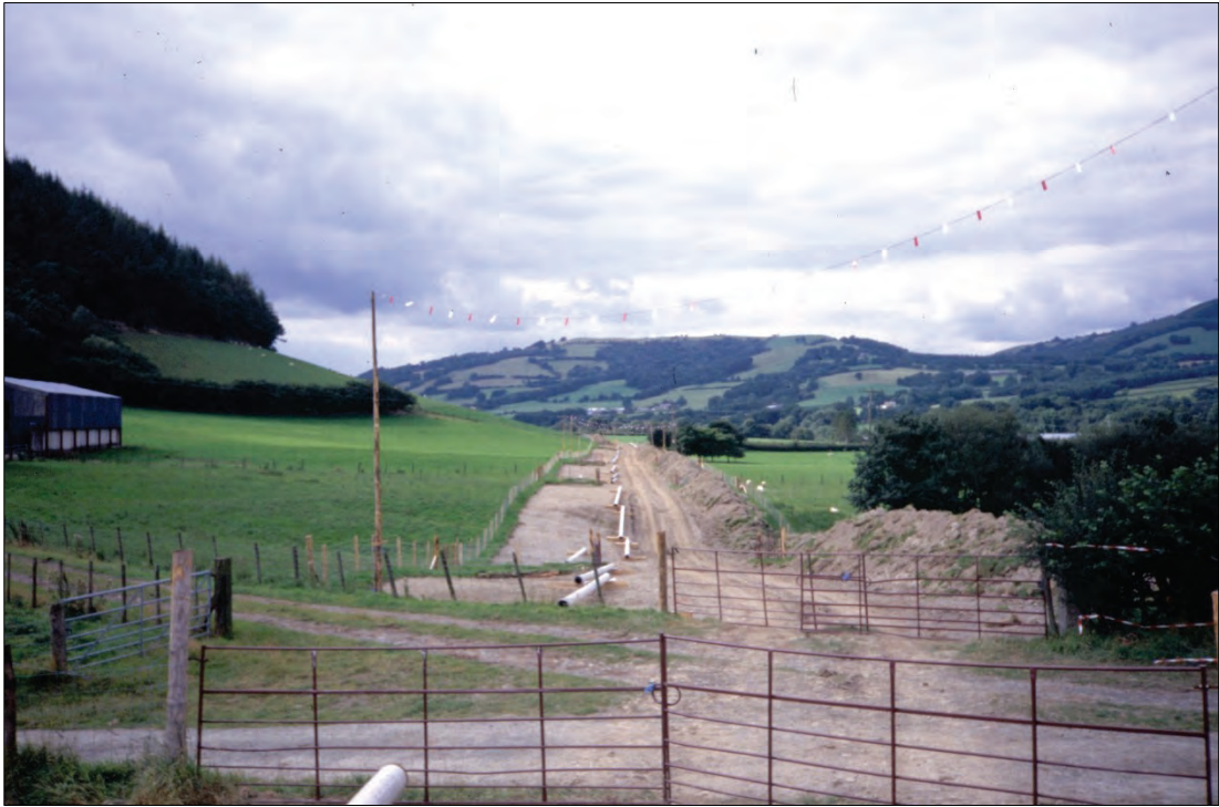
Figure 5-3: Typical Pipeline Stringing
