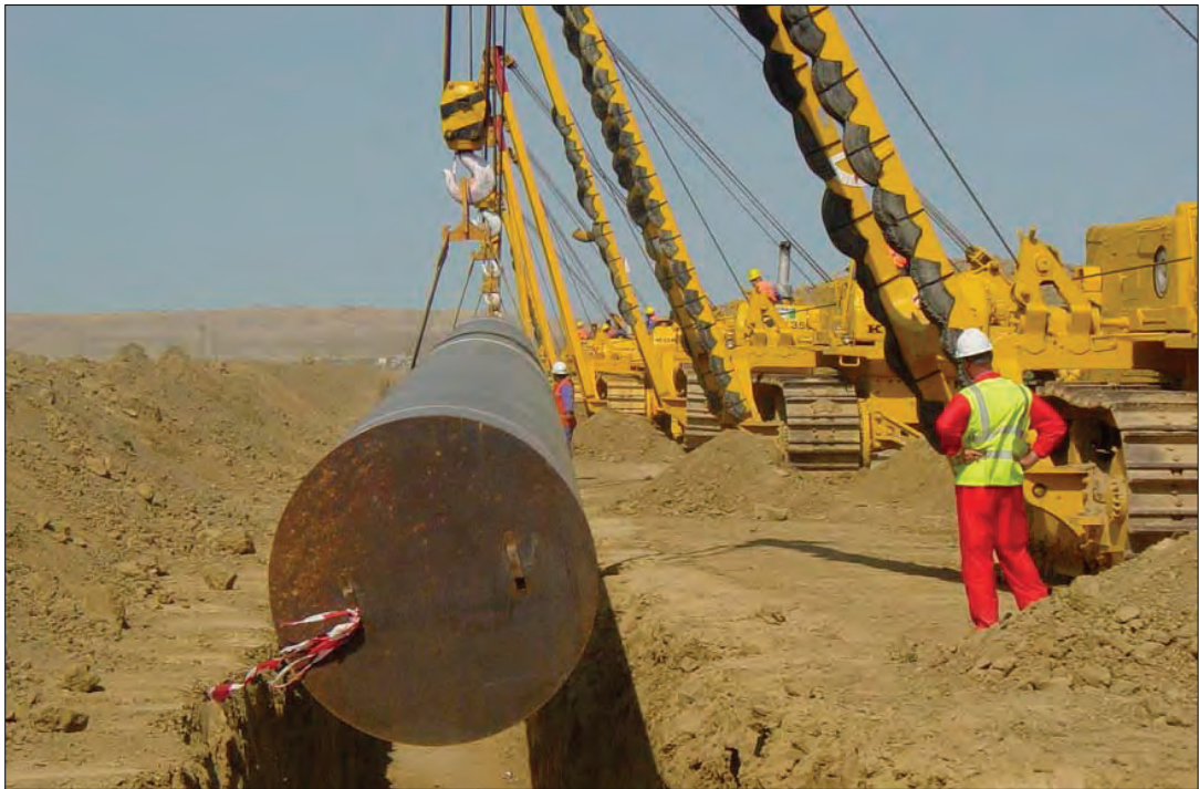
Figure 5-6: Lowering-in of the Pipeline
